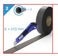
Measure the circumference of the service penetration and cut the Multiwrap to size with a knife. Remember to keep an extra length of at least 10 mm to create an overlap.
