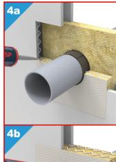
Seal the remaining recess with Multimastic SP or with the Multimastic C System or Multimortar System.
