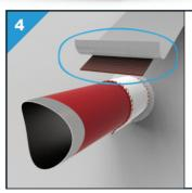
Remove the protective film at the back and wrap the Multitherm Bandage around the service penetration. Make sure that the closing side is at the bottom of the service penetration and that the Bandage has a minimum overlap of 10 mm. Press everything down firmly.
